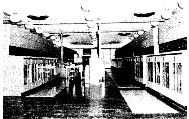
31.31 Figure 10-40.— Automatic relay center.
