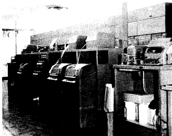
31.32 Figure 10-41. —Intercept section of automatic relay center.
